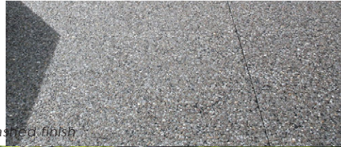
In-situ concrete with an exposed aggregate finish
