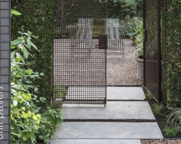
In-situ concrete with an acid washed finish
