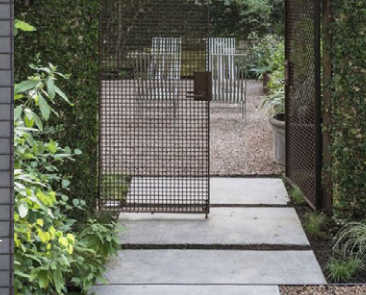
In-situ concrete with an acid washed finish
