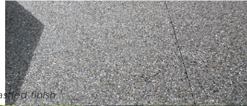
In-situ concrete with an exposed aggregate finish
