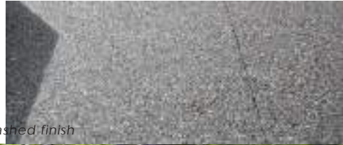
In-situ concrete with an exposed aggregate finish
