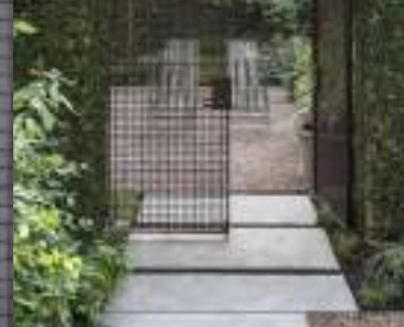
In-situ concrete with an acid washed finish
