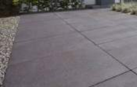
In-situ concrete with a coloured oxide added, and an acid washed finish
