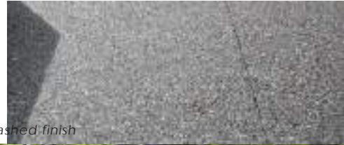
In-situ concrete with an exposed aggregate finish
