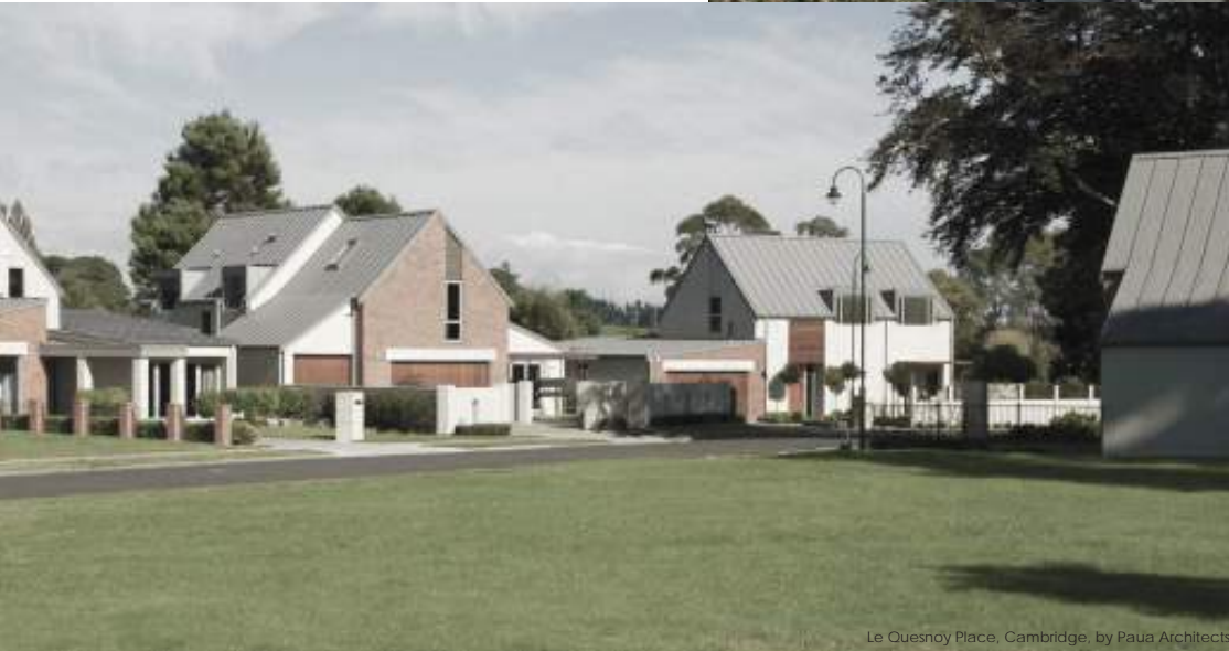
Le Quesnoy Place, Cambridge, by Paua Architects
