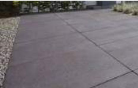
In-situ concrete with a coloured oxide added, and an acid washed finish
